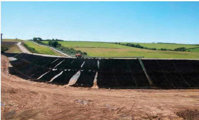
Geocell Panels positioned prior to fixing
