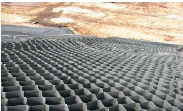
Geocell panels positioned and fixed prior to filling
